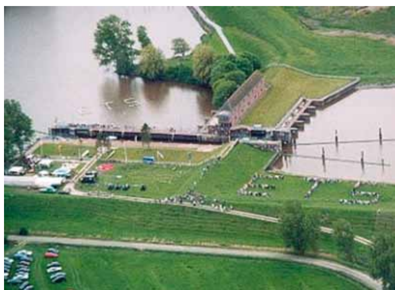
Figure 18: Aerial view of Nordfeld dam and weir
