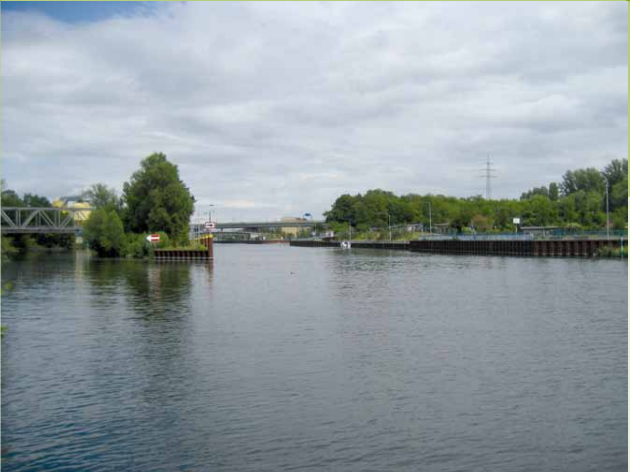
Figure 27: River Spree at the Charlottenburg sluice showing a shortened meander stretch and the channelised river bed
