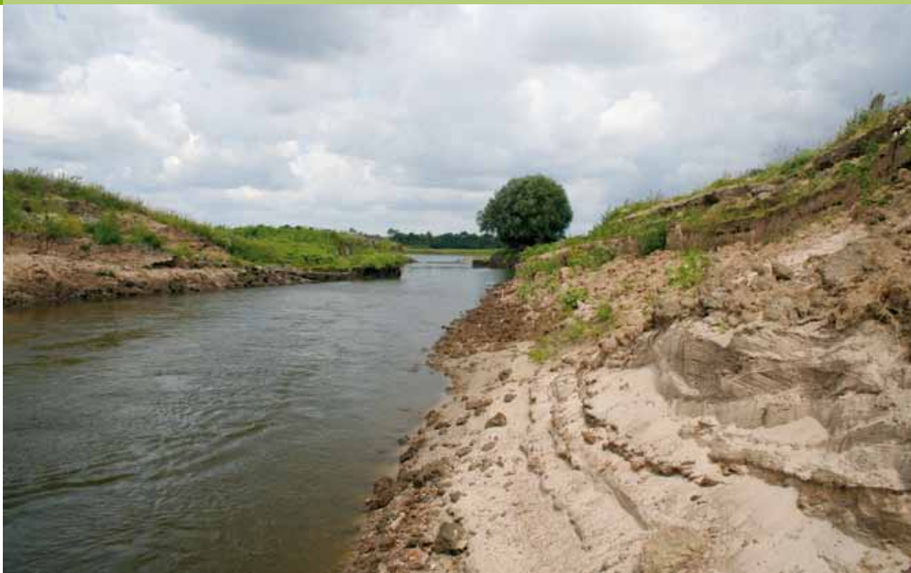
Figure 26: Compensation measure - construction of a side channel connected at mean water level in the Mittelelbe (middle Elbe) region near Magdeburg
