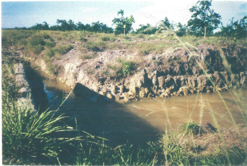
Pict. 9 Drainage channels in the TCC farm, with erosion of the banks of the channel visible
