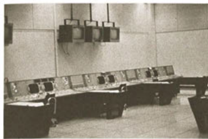
FIGURE 8: Vehicle systems staff support room.
