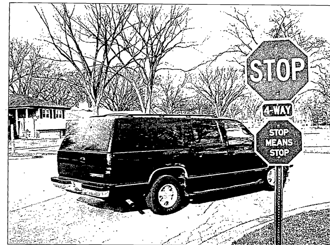
Park Ridge residents were complaining to the city that there were more rolling stops during the holidays so Public Works employees installed new signs, pictured above, at four intersections, Washington and Michael John, Weeg Way and Parkside, Vine and Belle Plaine and Thorndale and Canfield.
