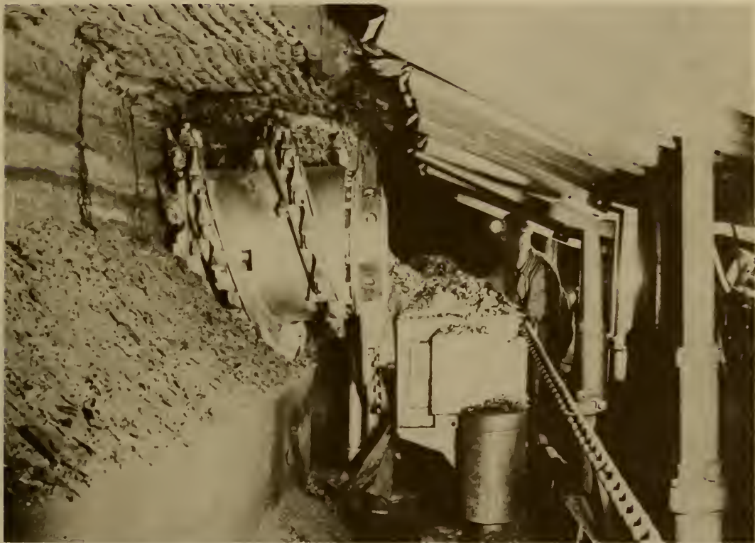
FIGURE 42. - Shearer loader making roof cut. (Courtesy Eickhoff-National Mine Company.)
