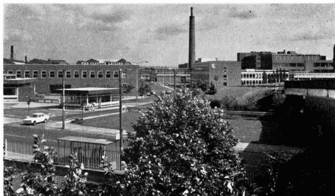
A view of the main entrance to the present site of the Clayton Aniline Co. Ltd, which celebrates its centenary this year
