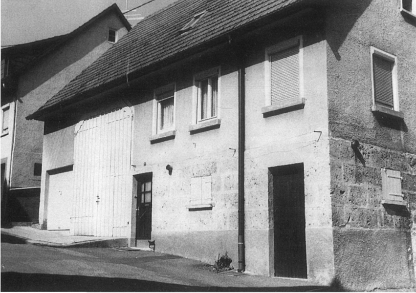
A smallholder's "Einhaus," with living quarters, barn, stall, and shed under one roof.
