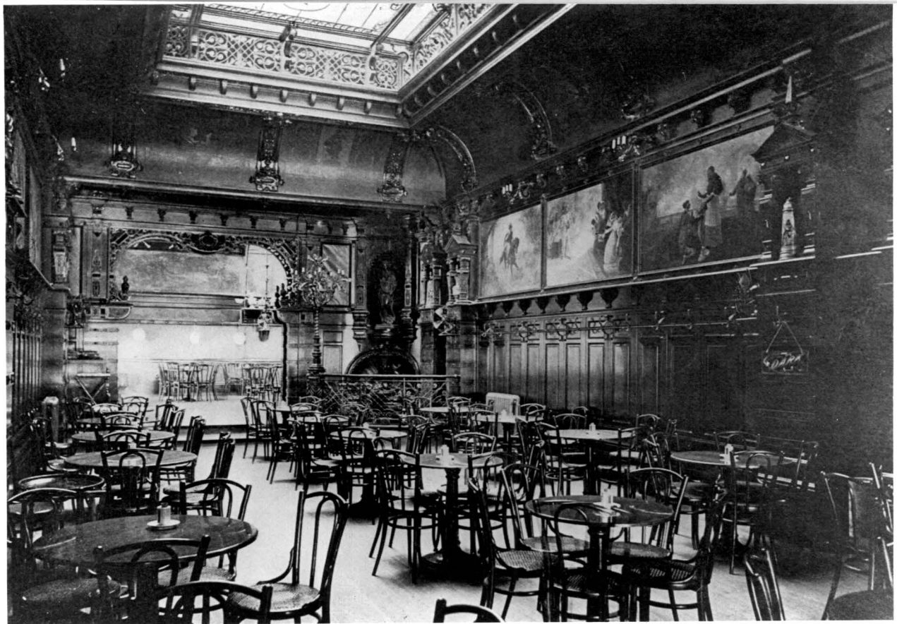
The front barroom, c. 1904
