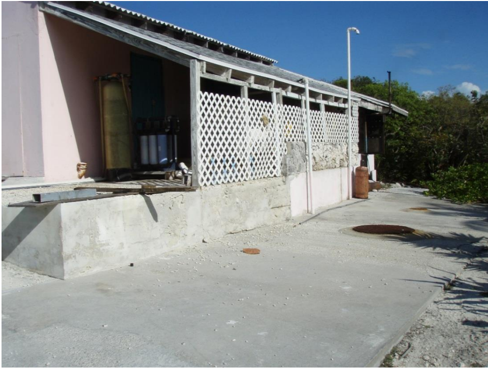
Photo 4-57. Exterior of Building Housing Reverse Osmosis Plant
