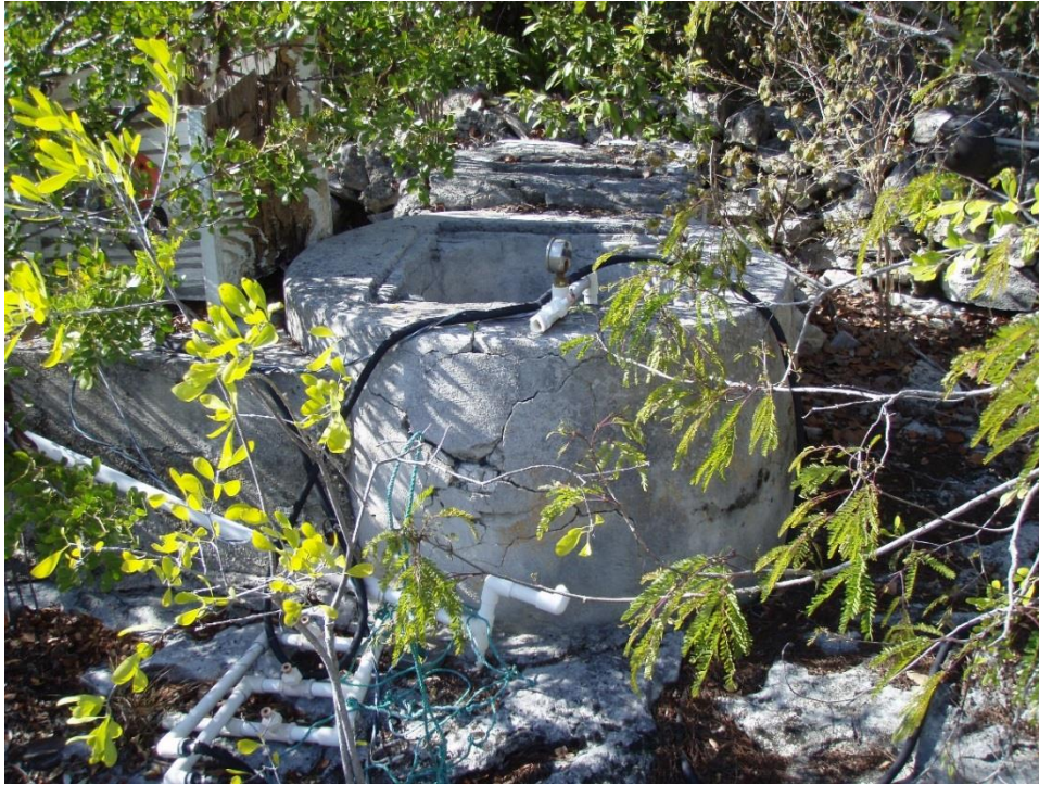
Photo 4-62. Abandoned Well Structure at the Former Agricultural Area near the Marina Basin on Children's Bay Cay
