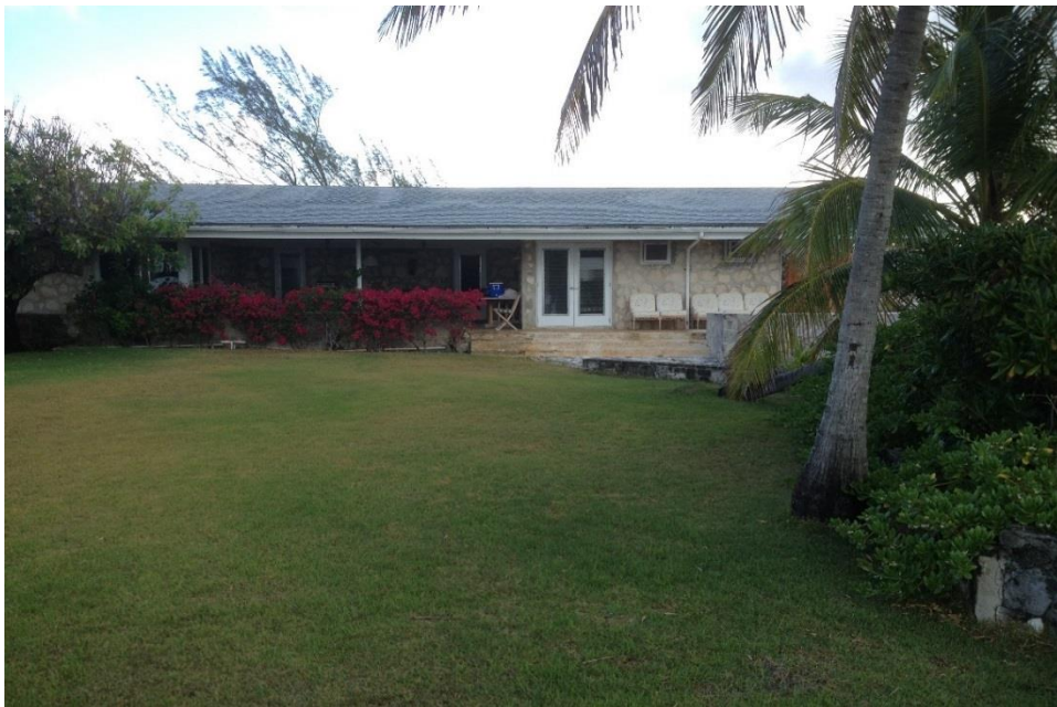
Photo 4-53. Main Residence on Children's Bay Cay
