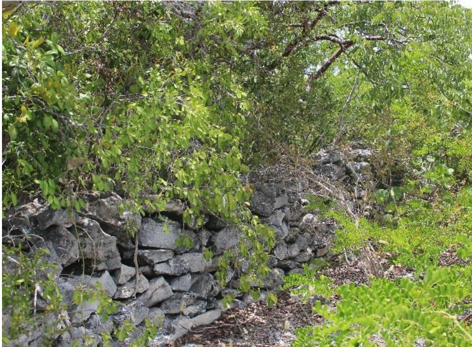
Photo 4-72. Dry Stone Wall – Children's Bay Cay
