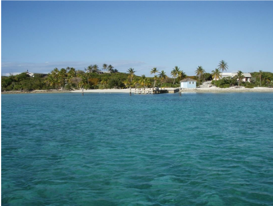
Photo 4-52. Existing Development on Children's Bay Cay as Viewed from South Side of Island. Residence and guest house on hilltop to left, pier and waterside storage in center, diesel-powered generator and RO plant in buildings behind coconut trees on right.
