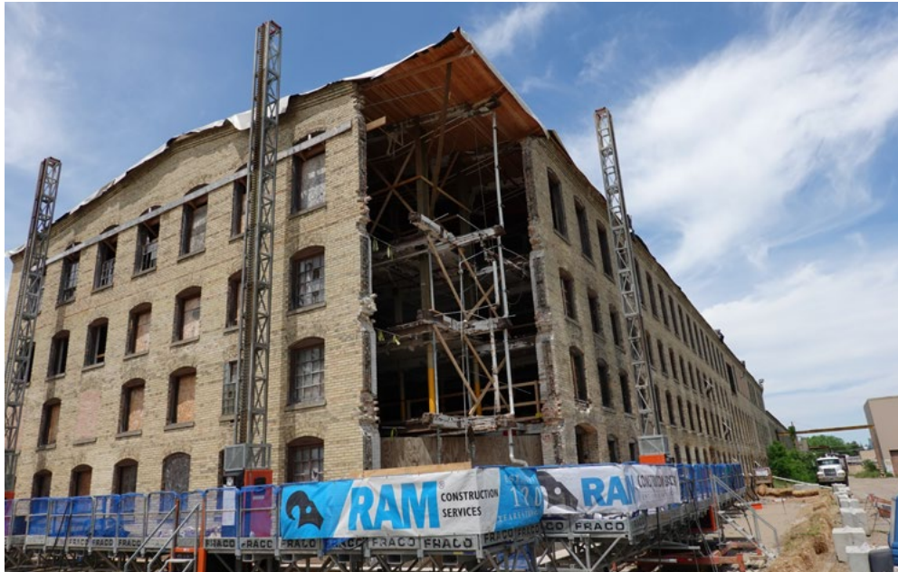
Corner of south east corner of brick building to be restored.
