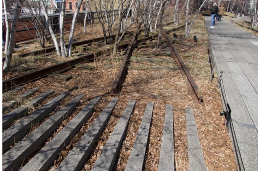
Ballast for railroad rails and allow a landscape of “volunteers” to grow between the track over time suggesting the abandonment of the rail line. Shown here are paper birch trees on the Highline in NYC.
