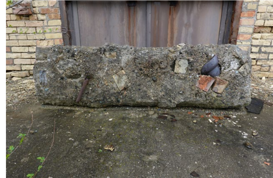
Existing Mill concrete conglomerate with embedded rubble and bottles.
