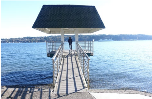
Here, a structure on Sinclair Inlet in Bremerton, WA, is an unintentional sonic listening pergola. When a visitor stands within the roof structure the wave action is reflected up and into the pergola. A parabolic reflector would have been more effective at capturing the phenomena.
