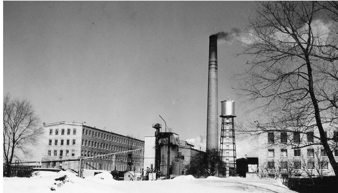
Historical image and model of original coal plant smoke stack.
