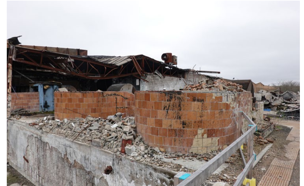
Image of future rubble consisting of glazed tile, CMU "cinder block" and cast concrete block each of these building texture will provide a variety of surface texture and color when added to another project rubble.
