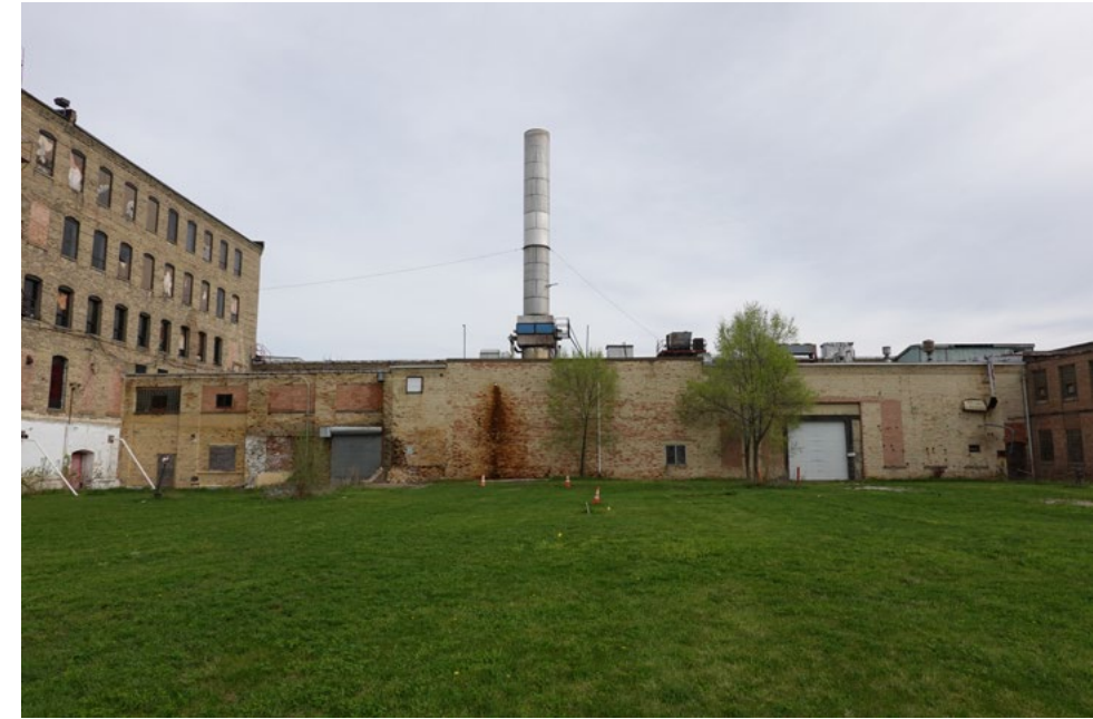
Exterior of existing stainless stack.
