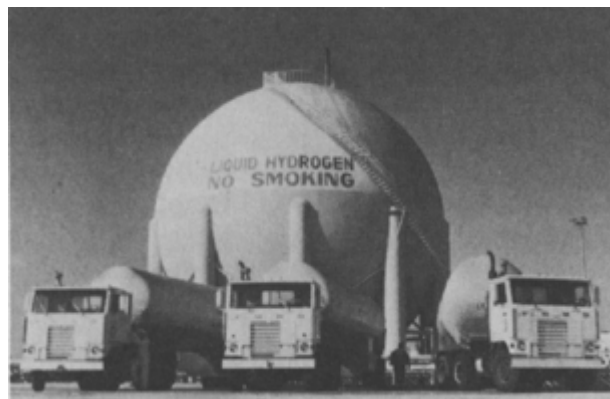
Abb. 35: 3800 m 3 LH 2 Speicher am Kennedy Space Flight Center in Florida (Photo NASA)
