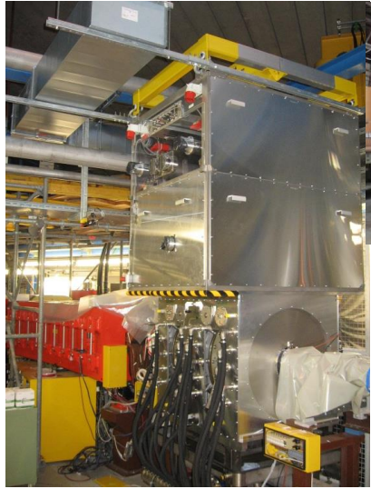
Three new MA acceleration cavities installed (50 kV, h=2) and power converters
