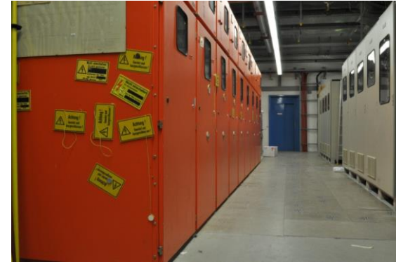
Replacement of main dipole power converter (for 10 T/s, 50 MW)
