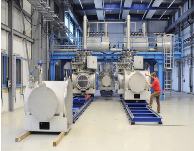
GSI: Series test facility for the SIS100 s.c. dipole magnets, string test, current leads and local cryogenics components.
