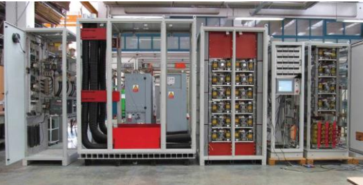
Three new MA acceleration cavities installed (50 kV, h=2) and power converters
