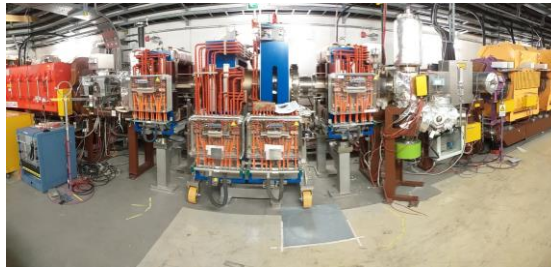
SIS18/SIS100 IPM monitor system manufactured and installed
