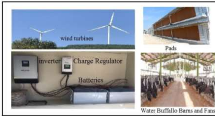
Figure 1. Water buffalo barns, wind turbine system and elements of ventilation and cooling systems
