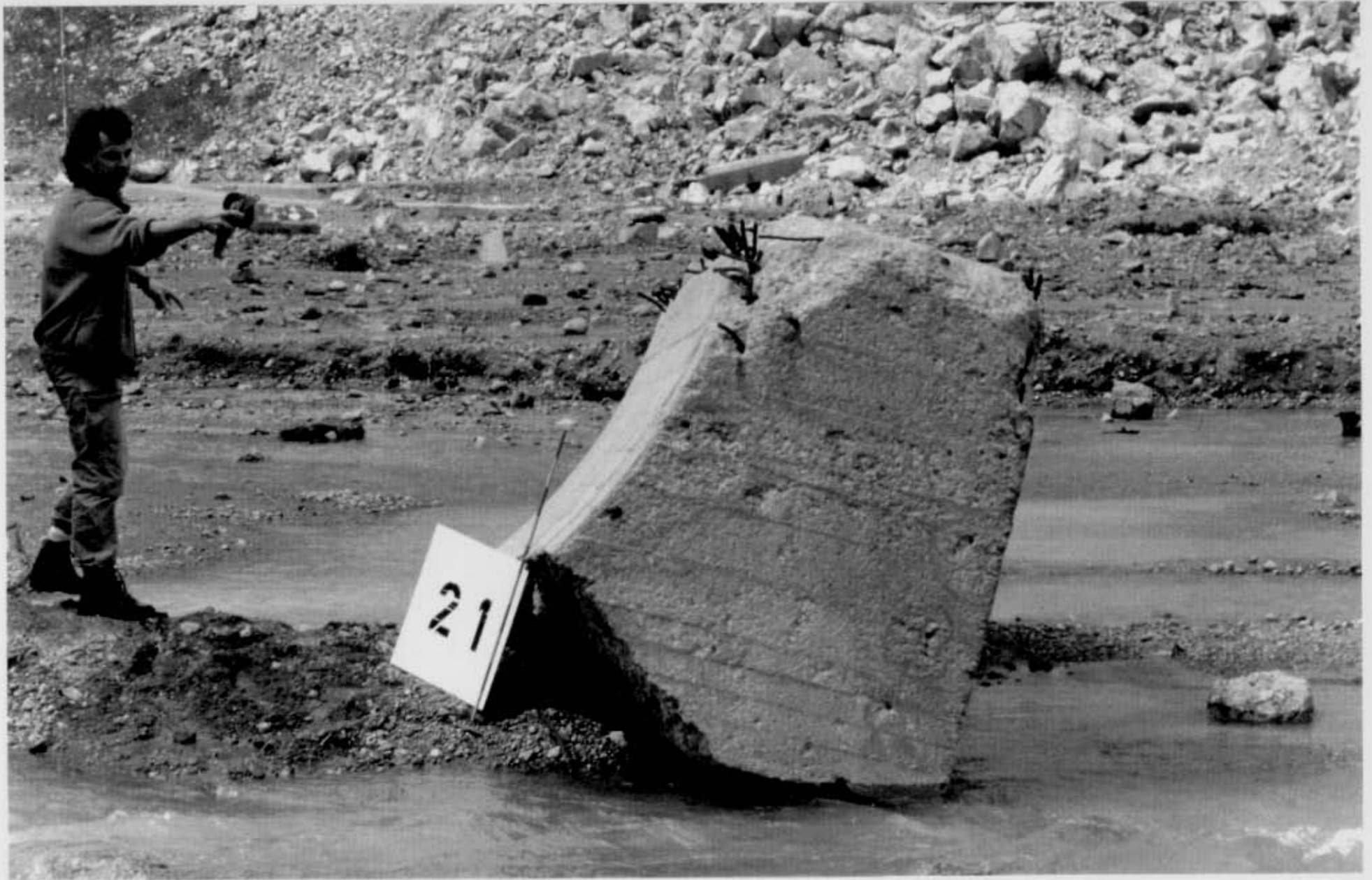
Concrete Block from Entrance Building Weight 15 tons, 370 m from Original Place
