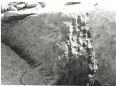
b) Original chisel marks on column base 4
