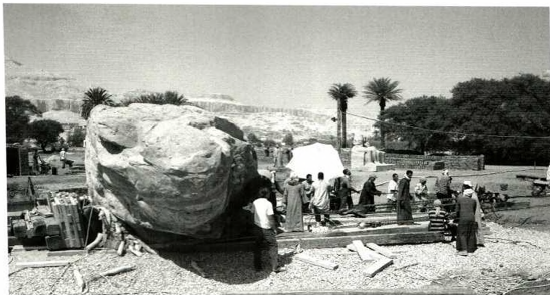
b) Moving the torso of the northern colossus on sledge, with two winches and air bags
