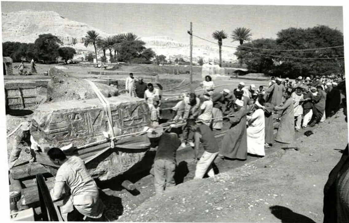
a) Moving the block of the plinth with the right foot of the northern colossus
