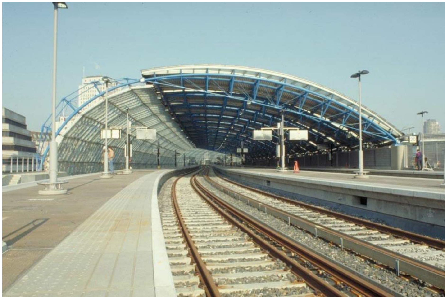
Sir Nicholas Grimshaw (Arch.), Anthony Hunt (Eng.): Waterloo International Terminal, London UK, 1993
