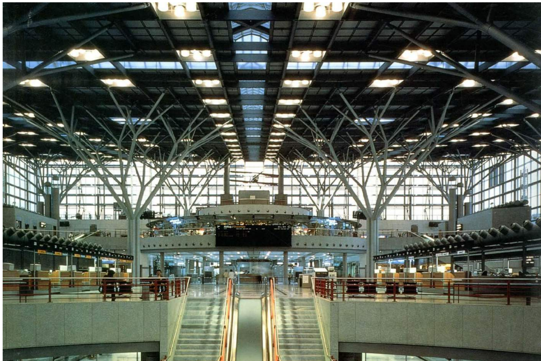
Gerkan, Mark & Partner, Schlaich Bergemann: Stuttgart Airport Terminal 3, 2004
