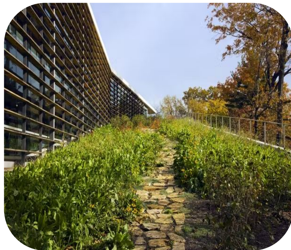
Photo of the CGC green roof in 2009 after its installation.
