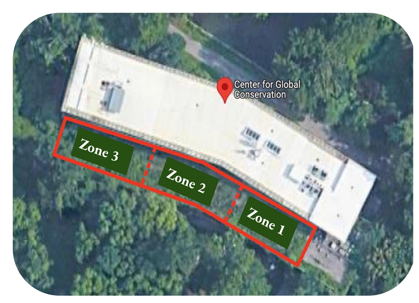
A satellite image of the CGC Green Roof with labelled zones.
