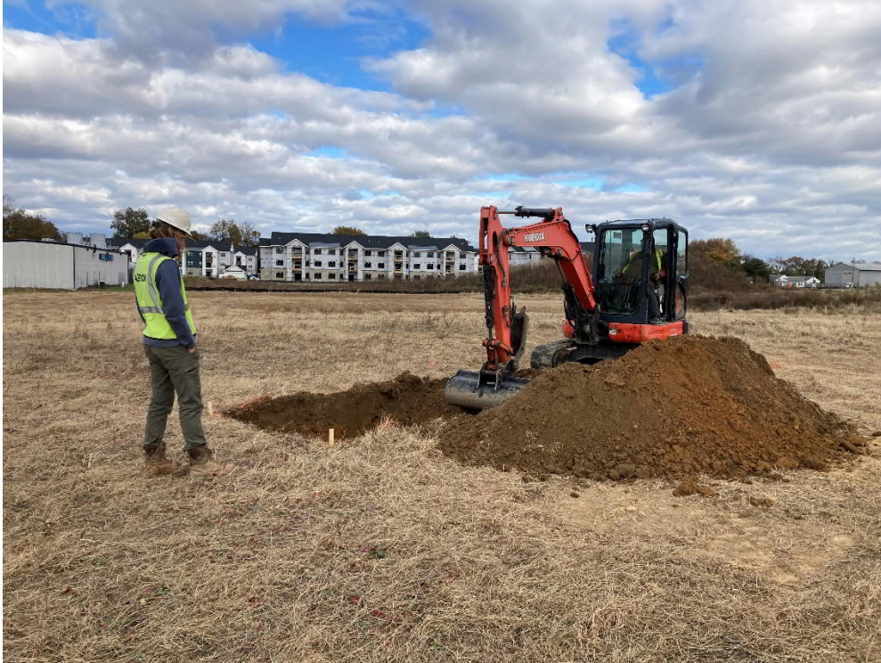
Photograph 4.8: Excavation of Strip Trench 2 in progress.
