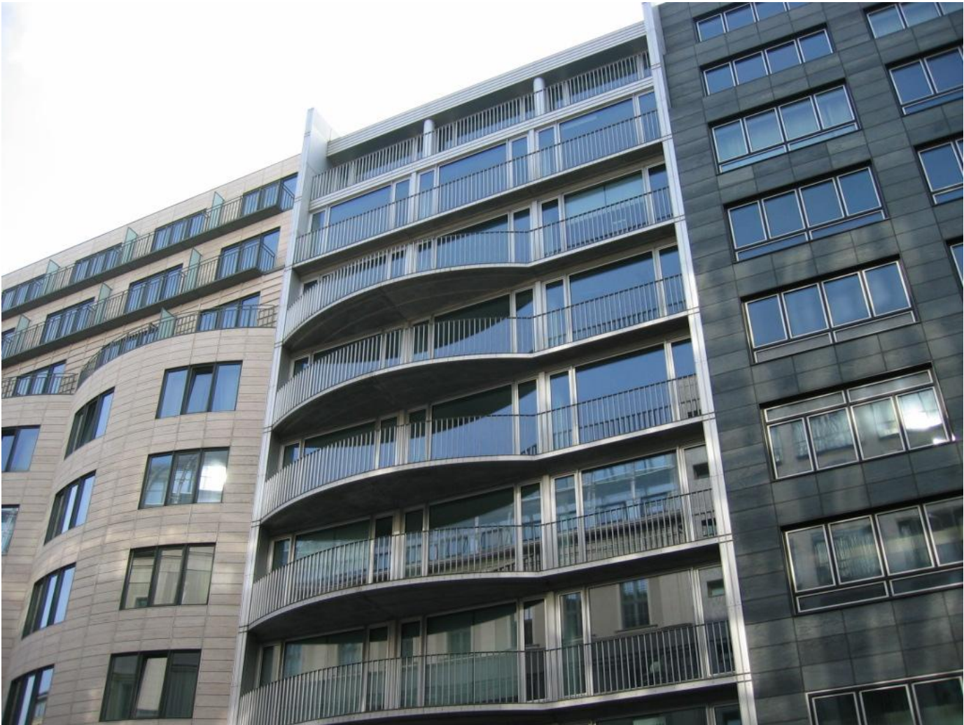
Figure 14. Atelier Building, designed by Josef Paul Kleihues.
