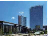
Beijing FA Center MITSUBISHI ELECTRIC AUTOMATION (CHINA)LTD.
