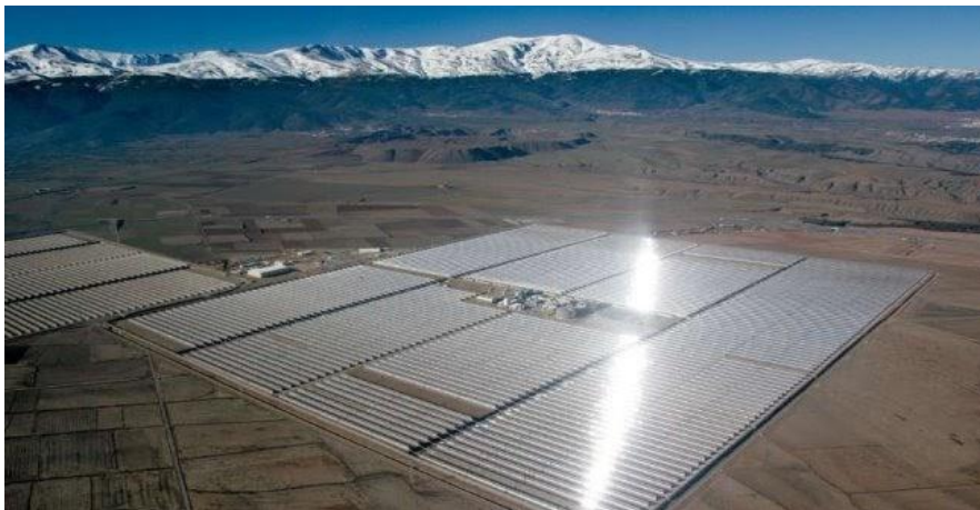
Image 2. Set of parabolic through arrays in Andasol 2 [6]
