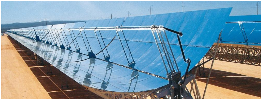
Image 1. Parabolic through. Andasol 3. Southern Spain. [4]
