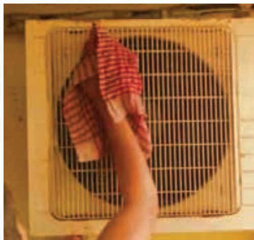
Fig. 4.5.3.4 : Cleaning of outdoor unit
