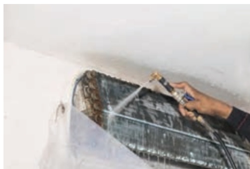
Fig. 4.5.3.7 : Cleaning the indoor unit
