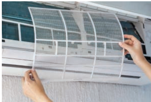
Fig. 4.5.3.1: Taking the filter out
