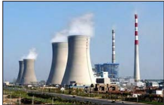
Fig. 4.6.1.3 Thermal Power Plant
