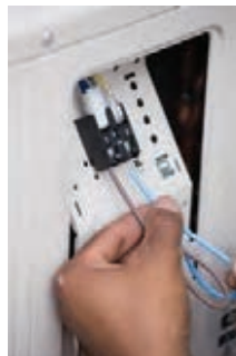
Fig. 4.4.3.10: Connecting electric wires
