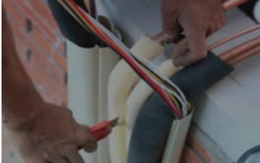
Fig. 4.4.3.13 : Wrap piping joints with insulating tape
