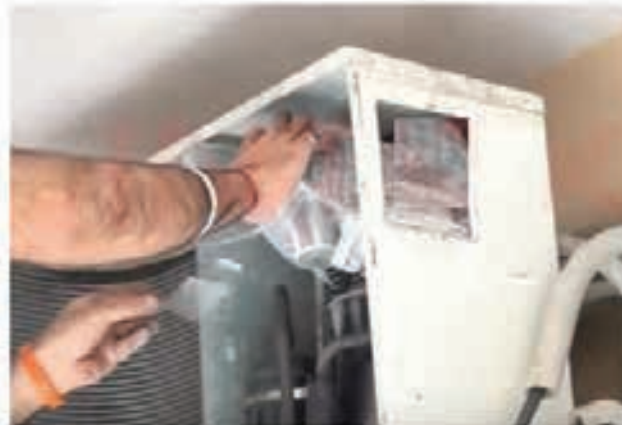
Fig. 4.5.3.12 : Covering the connection box
