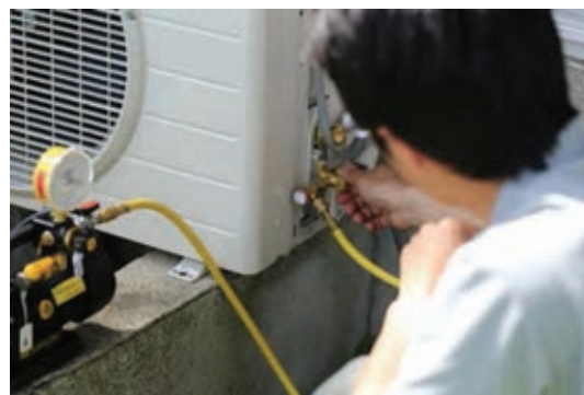
Fig. 4.4.3.12: Remove air and humidity
