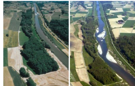
Sections of the River Thur near Niederneunforn (Switzerland) before and after river restoration. Copyright: BHAteam Frauenfeld
