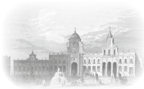
The Central Post Office of Chile
