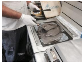
Figure 10 – Preparation of sealing compound
