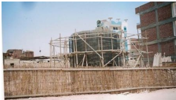
Photo 28: Construction of El-Hallous Pump Station
