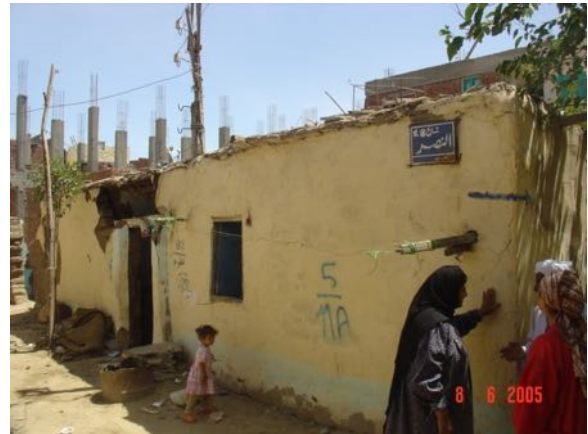
Photo 8: Buildings with temporary roofs
