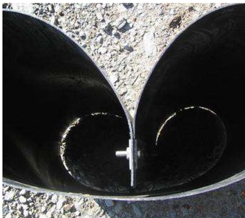
Barrier ends clamped together pointing in.
