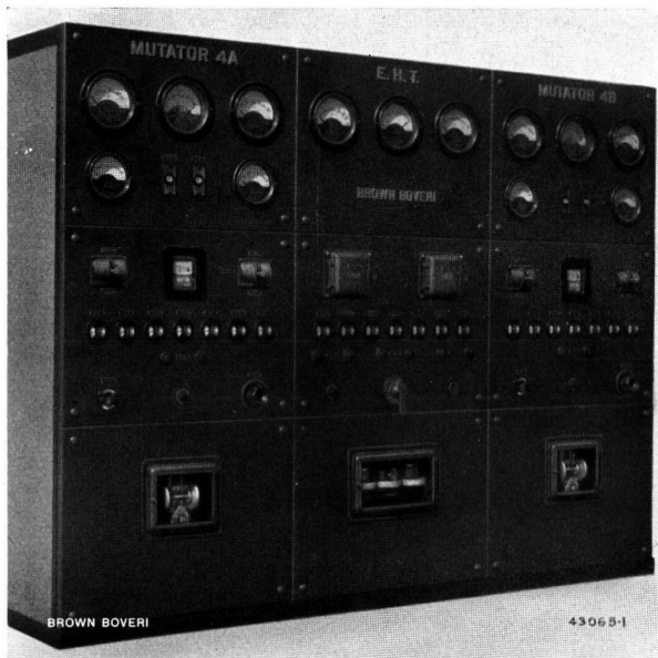
Fig. 12. — Warfield mutator switchboard — 1935 design.
