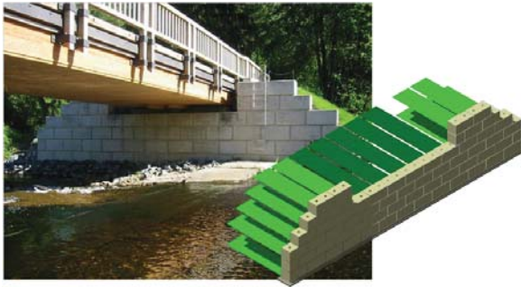
Fig. 8 Bridge abutment “Mandelholz “
