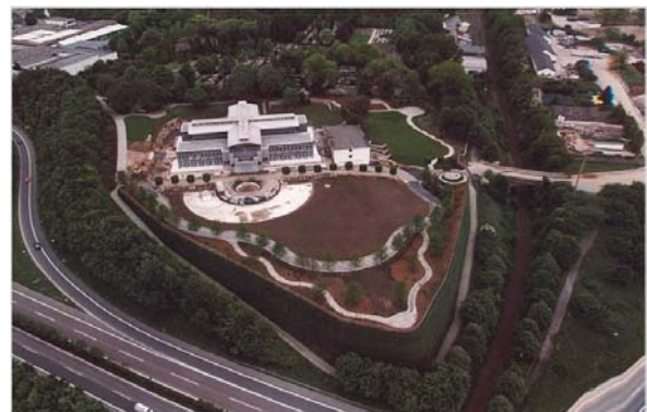
Fig. 12 Reinforced slope “Iserlohn I”
