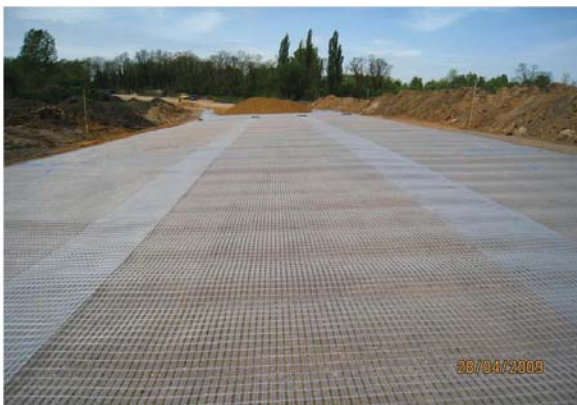
Fig. 9 Overbridging system “Hohenmölsen”
