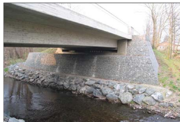
Fig. 7 Bridge abutment "K1355 near Ilsenburg"
