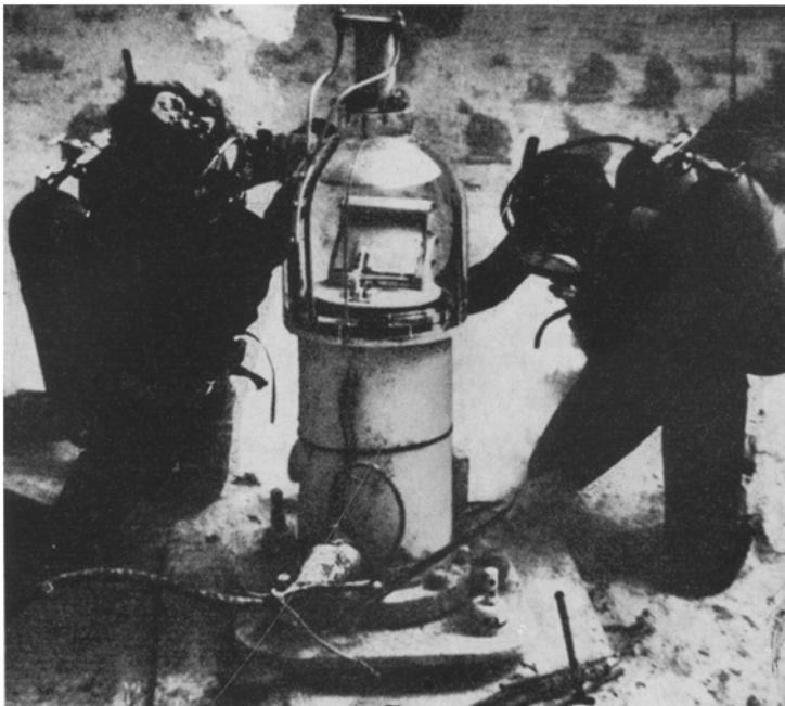
Fig. 8: TV camera with remote-controlled pan and tilt for recording activity of sharks. (After MYRBERG et al. 1969)
