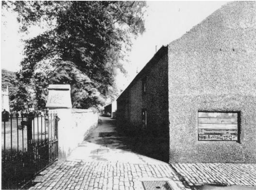
Rear of the almshouses next to the then narrow Bride Church Lane Courtesy © Crown Copyright. NMR Ref BB68/2067
