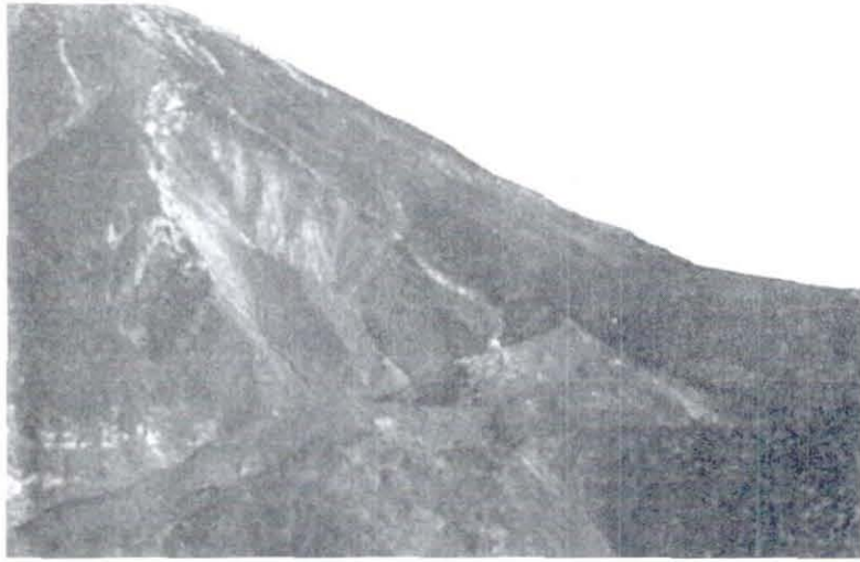
Photo 1 Large-scale Slope Failure at Southern Frank of Mt. Ontake
