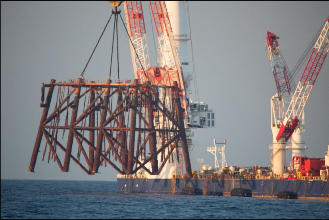
The top section of HI-A-389-A is lifted from the water in July 2018 by Nor Goliath . Photo: G.P. Schmah/NOAA
