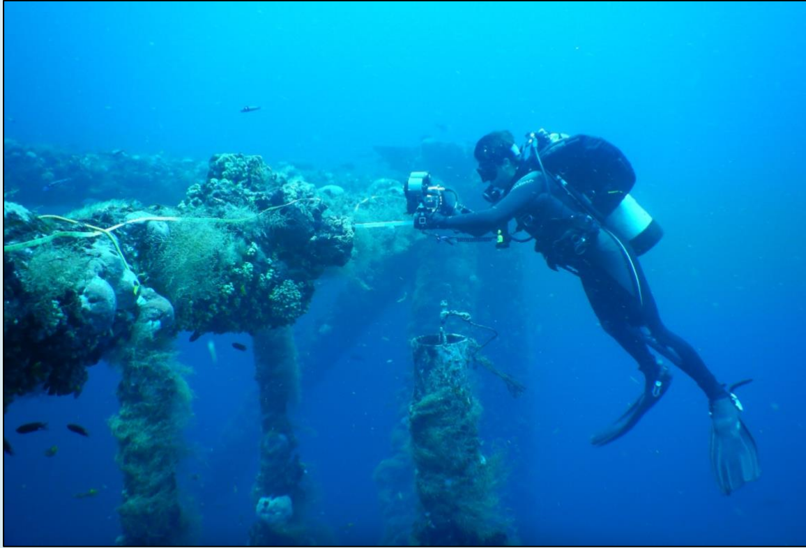
NOAA diver conducts a post-removal photographic transect on the outside of a horizontal support beam. Photo: Jimmy MacMillan/CPC
