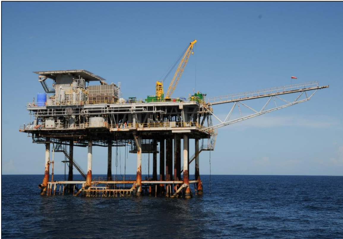
Figure 1.1. HI-A-389-A, an oil and gas production platform located in the northwestern Gulf of Mexico. Photo: G.P. Schmah/NOAA
