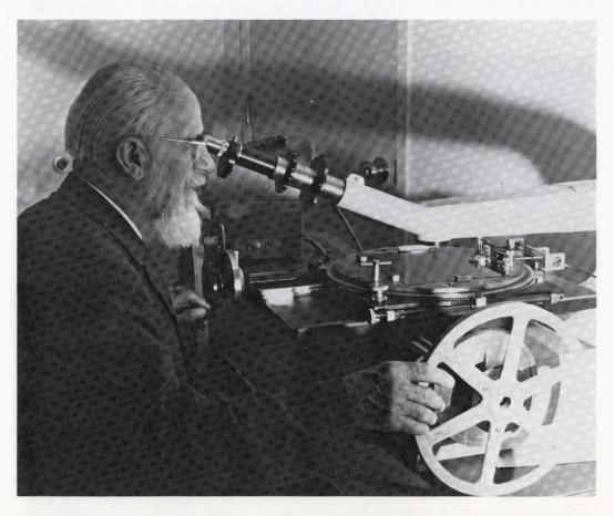
Figure 2: Dr. George Van Biesbroeck of the Lunar and Planetary Laboratory, University of Arizona, finding the accurate position of an image on a photographic plate, using a Mann Measuring Engine. (Courtesy R. B. Minton, Lunar and Planetary Laboratory, University of Arizona.)
