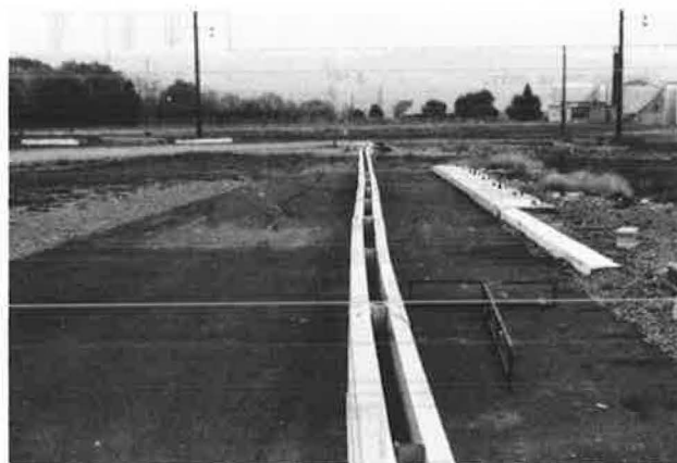
Figure 6. Median barrier that has 6-ft 3-in post spacing.
