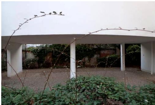
Figure 36 Space under the gallery, originally occupied by La Roche's bedroom (TB photo)
