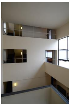
Figure 25 View of hall showing the alignment of the parapet of the upper corridor with the top of the big window (TB photo)
