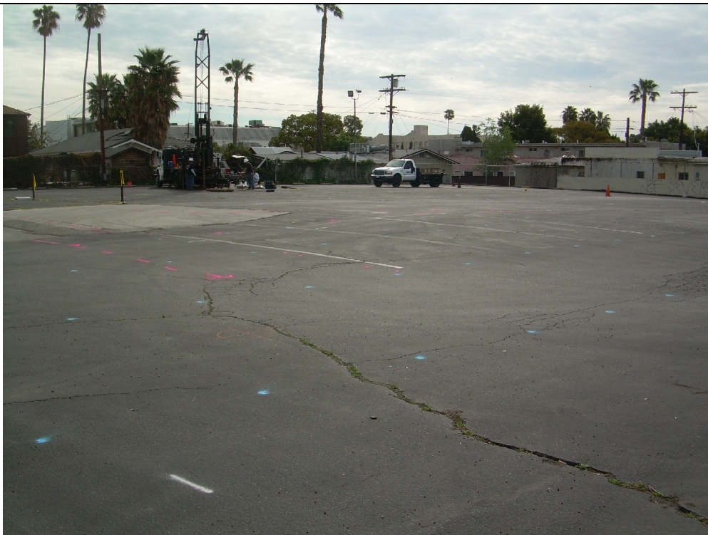
View southeast of the central portion of the Site.
