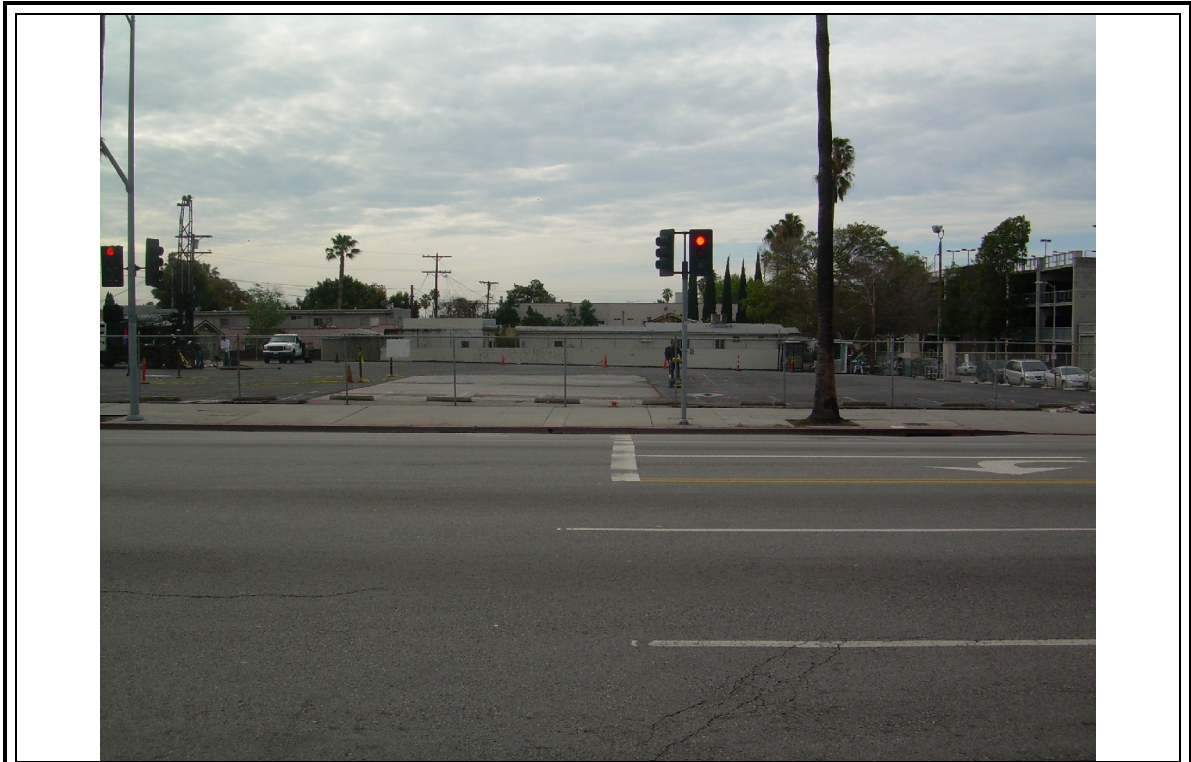
View south of the Site.
