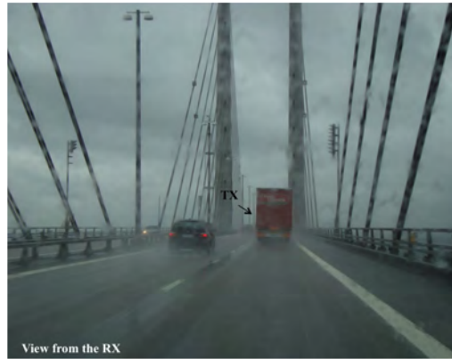
Figure 2.8: Measurement location for the on-bridge scenario.
