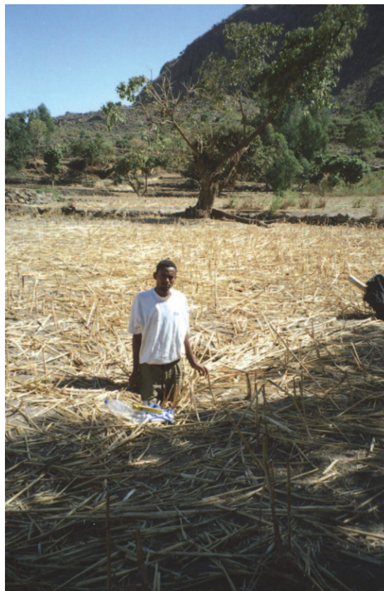
Fig. 13 Tensional cracks of en echelon type (up to 0.5 m wide) at the middle section of the large-scale landslide.
