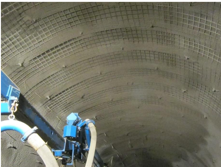
Figure 17: Spraying of shotcrete ribs
