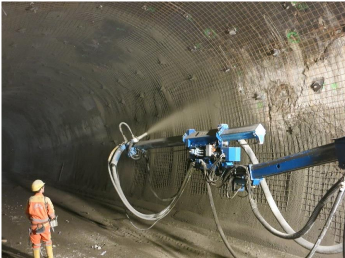
Figure 16: Shotcrete installation using manipulator
