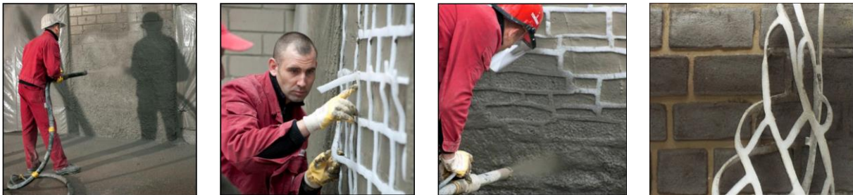
Figure 1-4: Steps to a shotcrete surface relief
