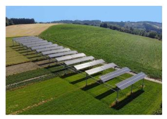
Figure 46: Agrivoltaic system in Heggelbach with 194 kW<sub>p</sub> capacity. © BayWa r.e.
