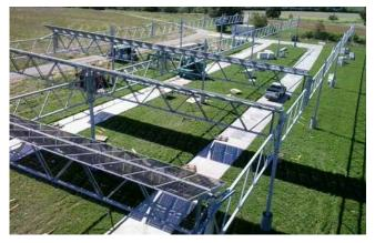
Figure 48: Construction roads to prevent soil compaction. © BayWa r.e.
