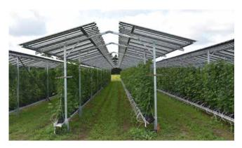
Figure 33: PV modules with spatially segmented solar cells and protective function in the Netherlands. © BayWa r.e.
