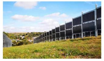
Figure 35: Bifacial modules installed vertically, Donaueschingen. © Next2Sun GmbH
