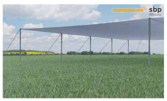
Figure 38: Semi-shade by tubular PV modules, installed between tension cables by the company TubeSolar. © sbp sonne gmbh
