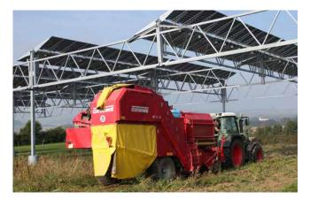
Figure 34: System with high mounting structure, permitting cultivation underneath the modules with the potato harvester. © Hofgemeinschaft Heggelbach
