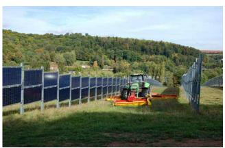
Figure 27: Vertically oriented bifacial modules in the Eppelborn-Dirmingen solar park, Saarland, with 2 MW<sub>p</sub> capacity, constructed by Next2Sun GmbH. © Next2Sun GmbH
