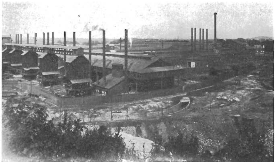
General view of Crystal City plant of the Pittsburgh Plate Glass Company.
