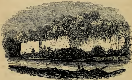
Fig. 29.—Great Wall at Copan.
