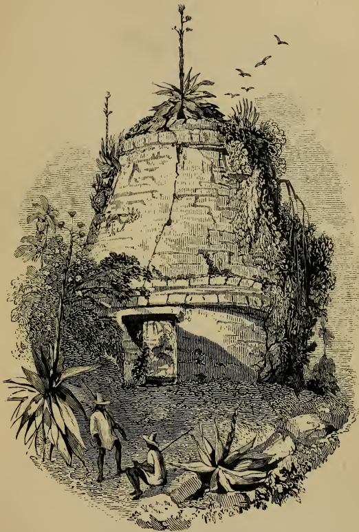
Fig. 35.—Circular Edifice at Mayapan.
