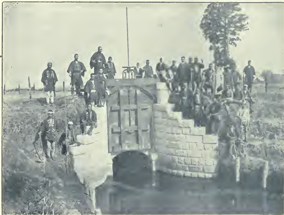
門樋造石坎ノ一台組水利通普水用田吉郡内河縣木枋 The First Flood-Gate of the Yeshida Irrigation Association, Kawachi District, Tochigi Prefecture.
