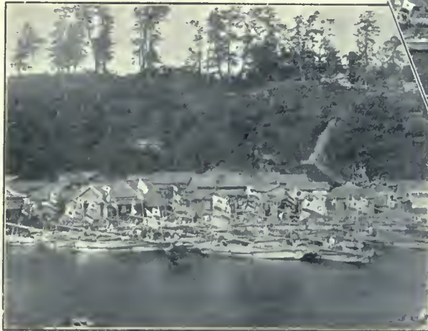
(160) Tsuruëura is known as a model fishing village. The villagers are engaged in fishing in distant seas, and their joint-savings at present amount to more than 10,000 yen. Every time war-funds have been raised, they have subscribed to the amount of 20,000 yen. Our views show how they look when they are ready to start on a fishing expedition.
