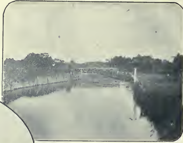
井渡掛合組利水通普路水用代沼見縣玉埼 The Elevated Aqueduct of the Minuma Irrigation Association, at Kawarabuki Village, Kita Adachi District, Saitama Prefecture.
