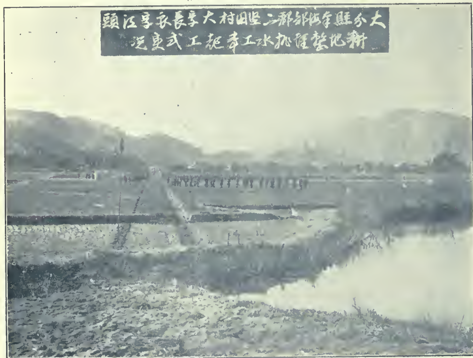
(179) Our view shows the commencement ceremony of the work of plotting and draining rice-fields at Shimo-Katada Village. The whole area to be improved was about 22 acres. The work cost over 2,400 yen and resulted in the creation of about 2 acres of fertile rice fields.
