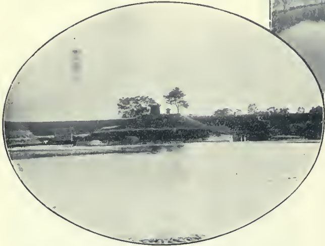
The First and Second Subterranean Aqueducts of the Same Association, at Suga Village, Kita Saitama District.
