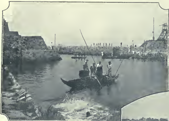
加古郡青年團二見支村ニ於テ見港ノ浚作業 Dredging Futami Harbor at Futami-Mura Branch, of the Young Men's Association of Kako District, Hyōgo Prefecture.
