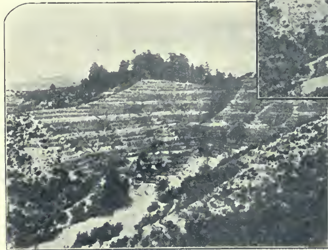
事工防砂ノ後工竣ルケ於ニ塚里一字町戸瀬 Landslides Prevented at the Same Place.
