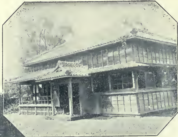
宮崎縣立圖書館外館 An Outside View of the Miyazaki Prefectural Library.
