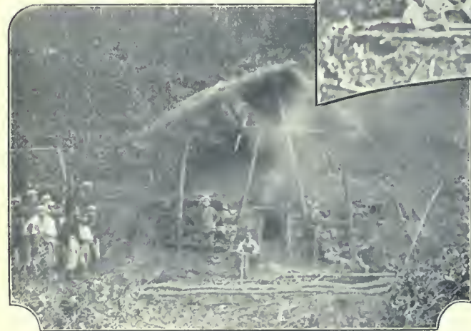
Our upper picture shows the charcoal-furnace mied with wood and ready to be burned. The furnace is made of stone and turns out about one ton and a quarter of charcoal at a time. The lower picture is an entire view of the furnace.
