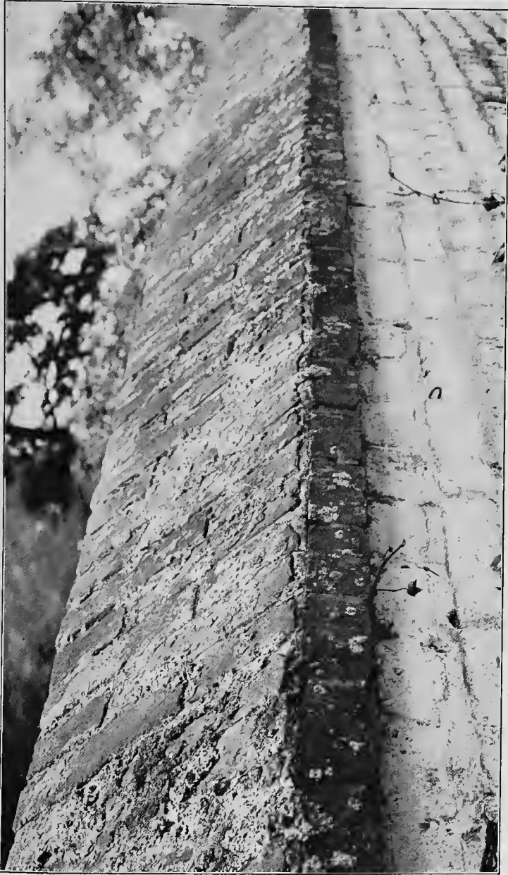
A SECTION OF THE LICHEN-COVERED GARDEN WALL
