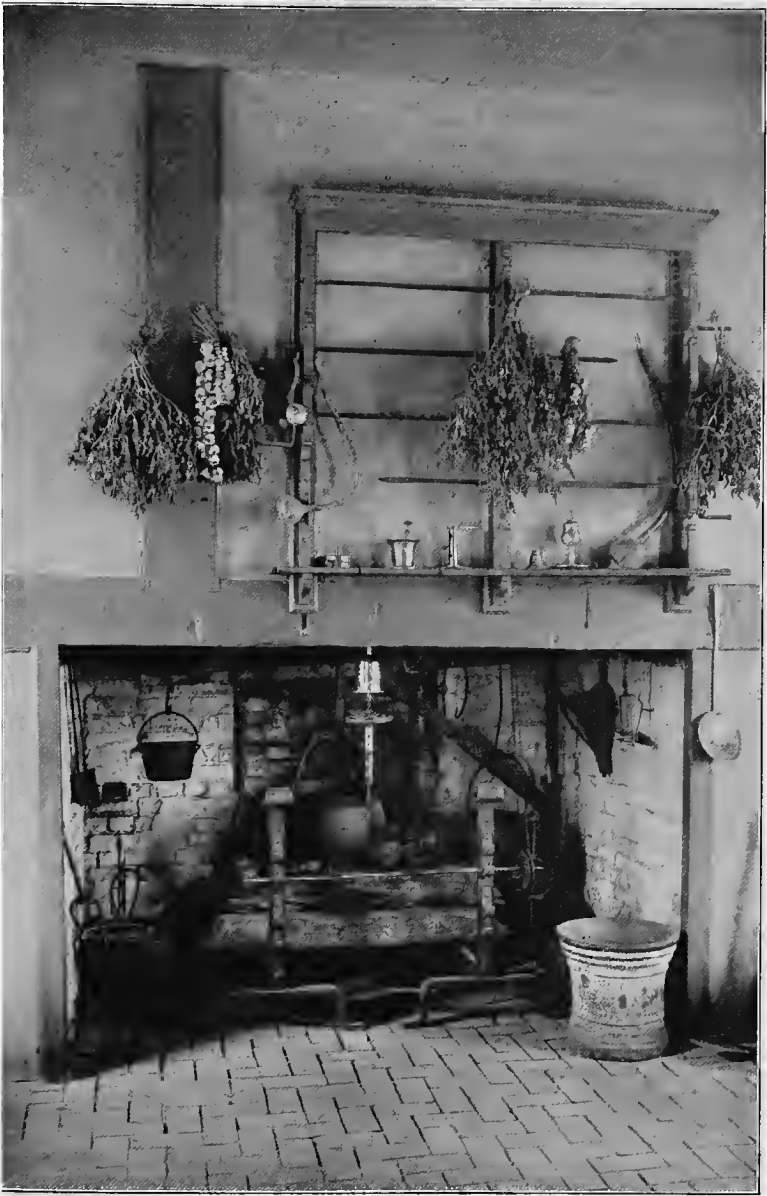
THE KITCHEN FIREPLACE
