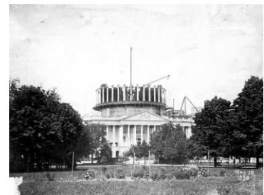
Dome Construction in 1858
