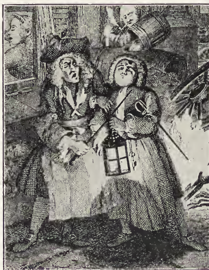
SECTION OF "NIGHT" BY HOGARTH SHOWING TWO MASONS
