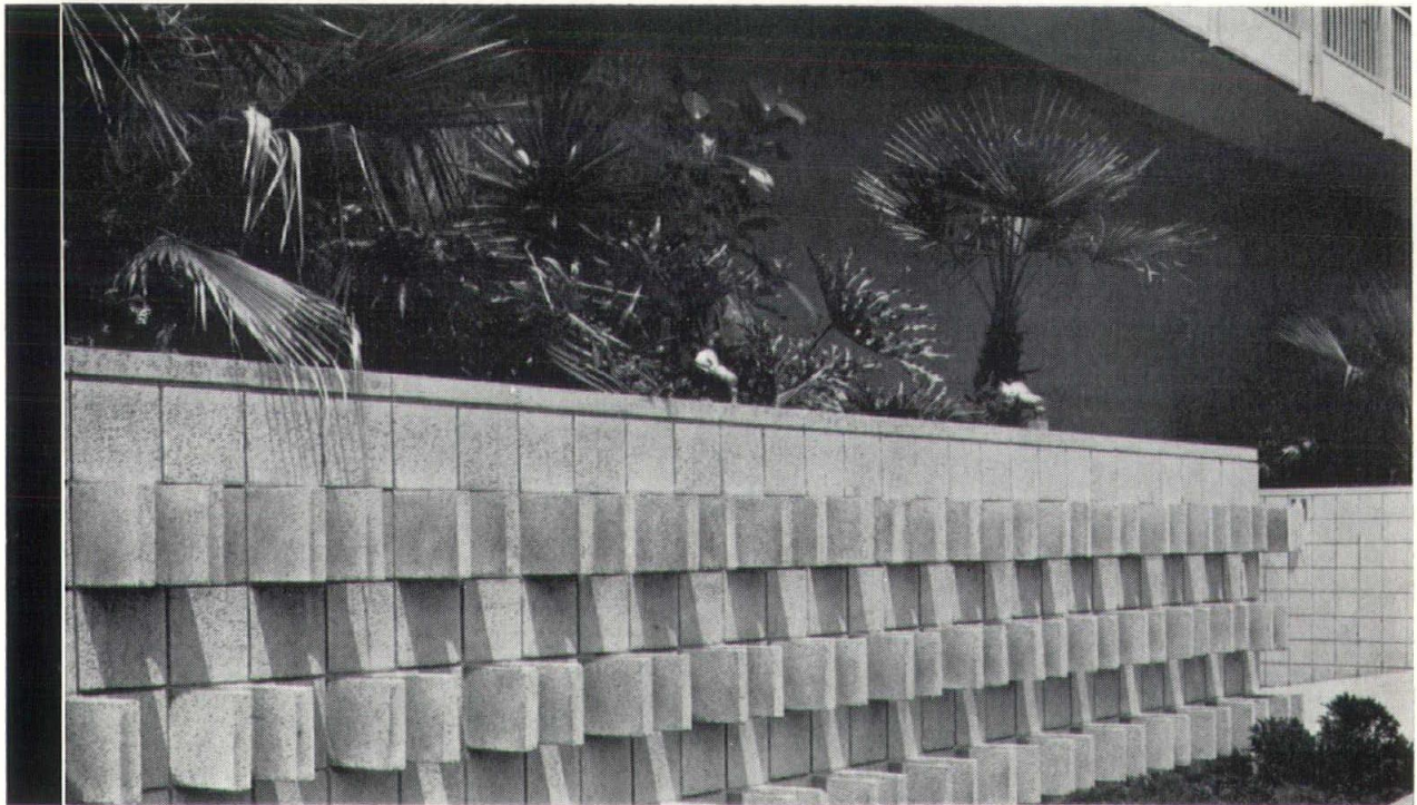
Here 8-inch square and lintel units create an unusual wall treatment.
