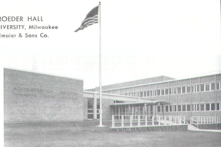
NEW ADMINISTRATION BUILDING MILWAUKEE SCHOOL BOARD Architect: Grassold-Johnson & Associates Assoc. Architect: Fred A. Wegner
