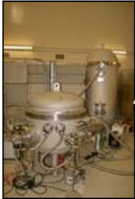
Deuterium/Hydrogen Storage tank
