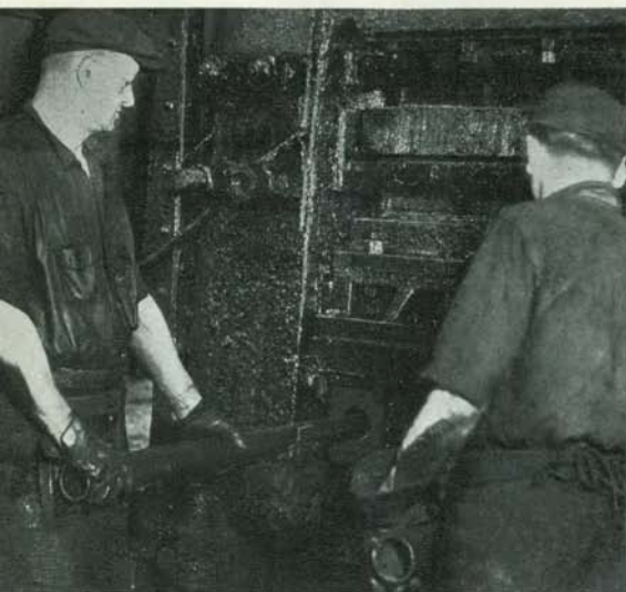
Tapering mechanical tubing at Monessen Works
