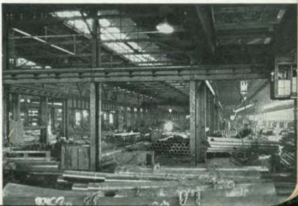
General view of Pilger Mill building at Allenport Works
