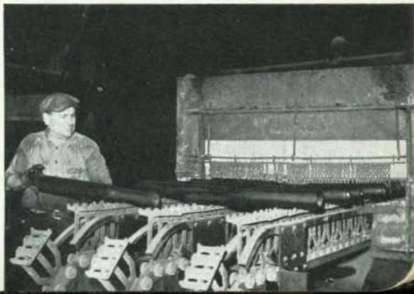
Bending pipe to specification patterns at Allenport Works
