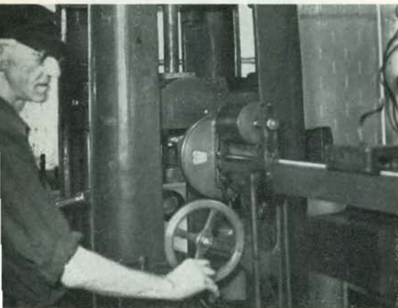
The tensile test. This machine is capable of exerting a 250,000-pound pulling stress.
