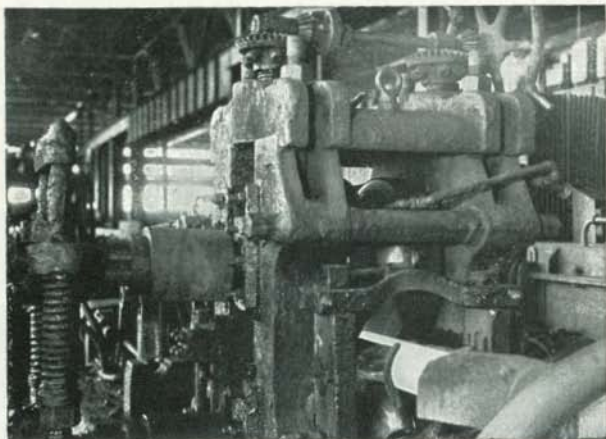
Sizing large pipe at the Pilger Mill.
