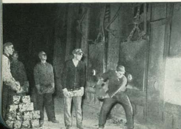
Charging an open hearth furnace with molten iron.
