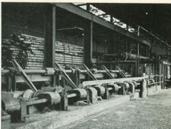
Pilger pipe leaving the normalizing furnace.
